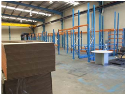
Work starts on the racking
