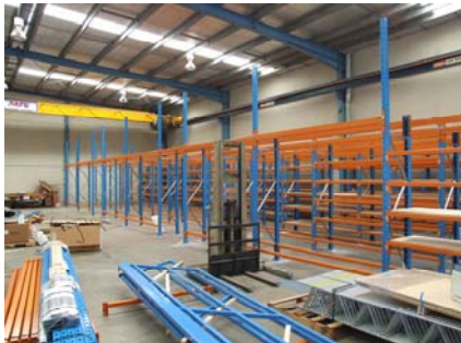
Racking Nearly Finished
